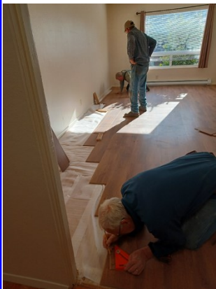
Both Councils led the effort to update the rectory for St Mary's in Coquille by removing the worn carpets and replacing it with laminate flooring. Participants were Brothers Ron McDowell (1261), Frank Roeder (17396) and Mike Hahn (17396).
